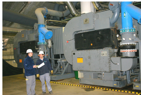
Figure 13: Energy distribution scheme and production plant with absorption chillers in Barcelona. (Source: Districlima, S.A.)
