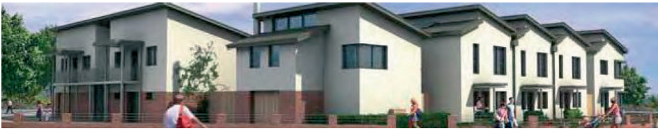
Figure 18: Greenwatt Way development, Slough, UK
