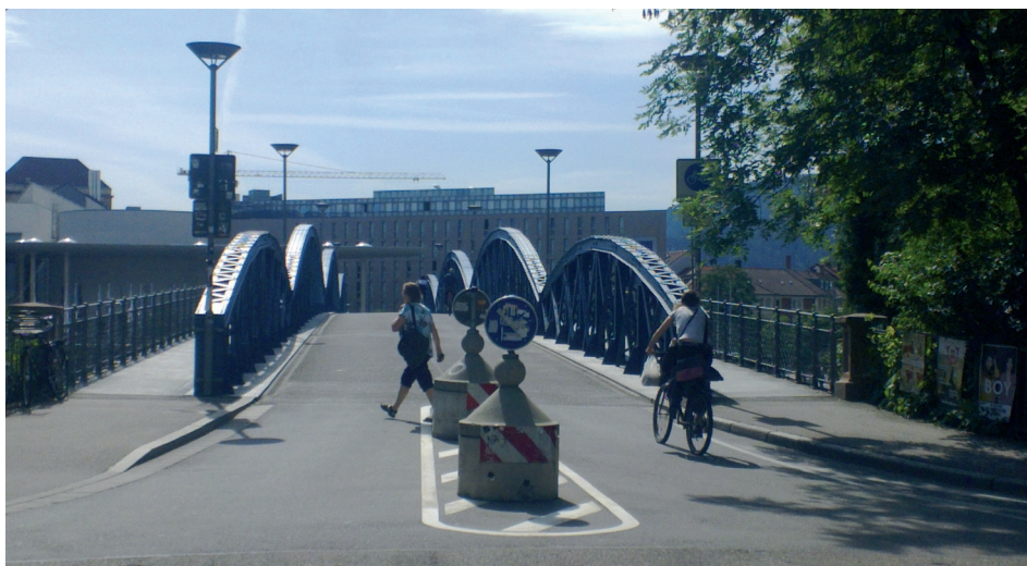
Figure 12: Cars do not have access to the bridge that is dedicated for bikes in the middle and for pedestrians on the sides. (Photo: A. Nuorkivi, Aalto PRO)
