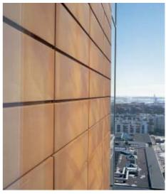
Cor-Ten steel, which was awarded the steel structure prize in 2000, has been used in both the frame and the details of the building.
